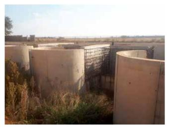
Reinforcing steel severely affected by rust
