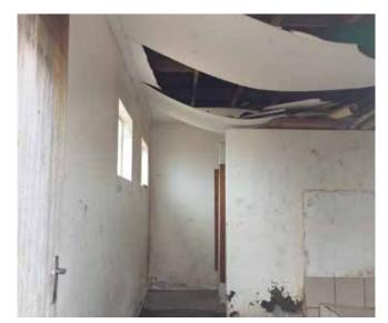
Blocked toilets and ceiling close to collapsing
