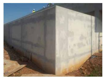
Lots of patched cracks on concrete
