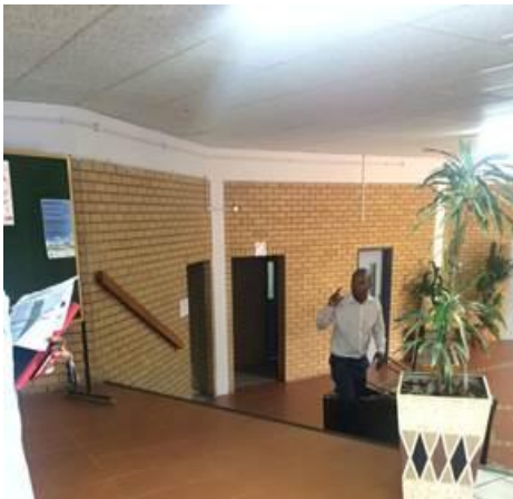
Picture 7: Inappropriate access to the 2 nd of two disability ablutions, due to poor planning during needs analysis, at CH Baragwanath Hospital (national facility)
