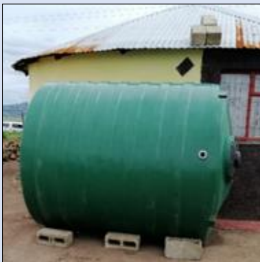
Water tanks placed on uneven surfaces without stays and stabilised with loose concrete blocks, damaging base of tank (left); a water tank that was not installed or in use was stored on its side and secured with a few loose blocks (right)
