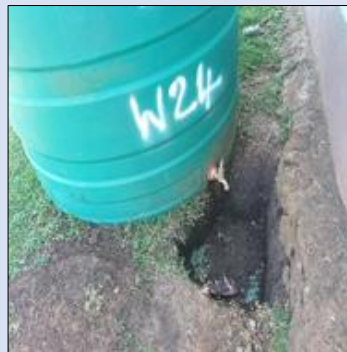
Inadequate material used as stays to secure water (left), water tank placed directly on ground with insufficient clearance between ground and tap (right), resulting in a hole being dug to facilitate water collection
