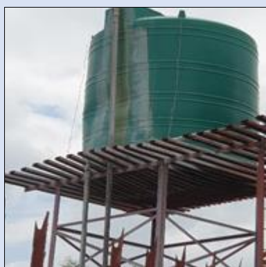
Bases of water tank stands were bent due to weight of water tanks when filled
