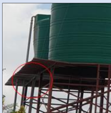
Bases of water tank stands were bent due to weight of water tanks when filled
