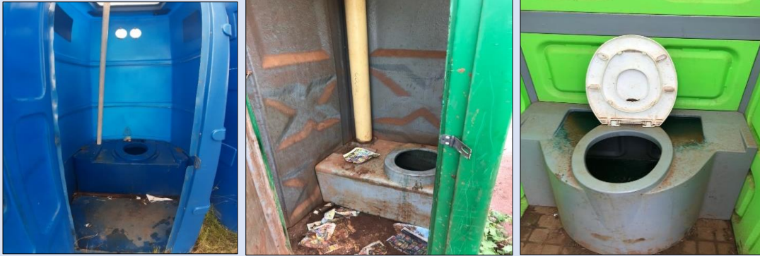
Toilets at Plot 30 in Kameeldrift and Zone 14 in Garankuwa that were not cleaned
