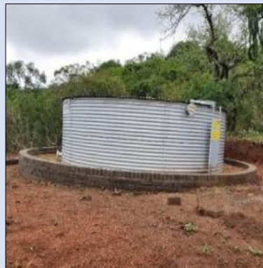
Kwambewu project: Pump house not completed (left) and piping not connected (inset); 28kl SBS tank not commissioned and surrounding fencing not completed (right).
