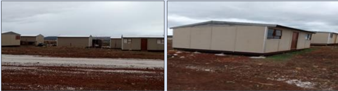
Temporary structures at KwanoNgoma in Jachvlakte
