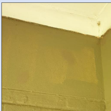
Paint was thinned and adequate coverage was not provided (left); Paint not cleaned after painting shower (right)
