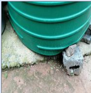
Water tanks placed on uneven surfaces without stays and stabilised with loose concrete blocks, damaging base of tank (left); a water tank that was not installed or in use was stored on its side and secured with a few loose blocks (right)
