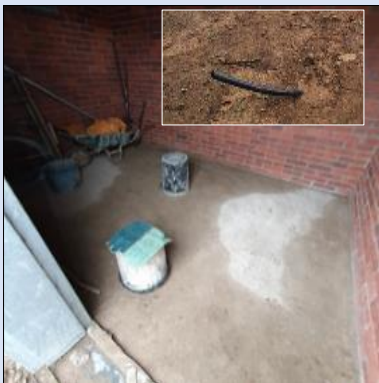
Kwambewu project: Pump house not completed (left) and piping not connected (inset); 28kl SBS tank not commissioned and surrounding fencing not completed (right).
