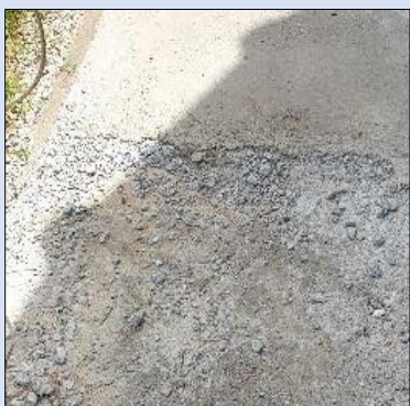
Poor concrete work around the rondavels (left); Cement not cleaned after installing shower doors (right)
