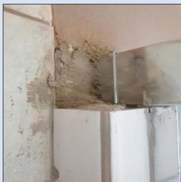
Poor concrete work around the rondavels (left); Cement not cleaned after installing shower doors (right)
